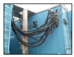
It will be important to ensure that the grounding system is reestablished after the unit has been refurbished. New 4/0 copper grounding will be installed for all new equipment enclosures.
