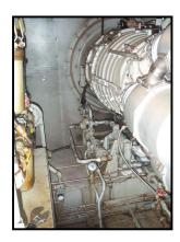
would be to consolidate the two pumps and fuel valve with a regulated fuel supply. The advantage of this alternate approach is a simplification of the system design and possibility the creation of some free space in the vicinity of the fuel day tank. To enhance the environmental conditions within the power trailer it will be necessary to modify the fuel day tank to include provision for containing a spill.
